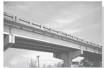
The prestressed concrete girders are simply supported and are used for this highway bridge.
