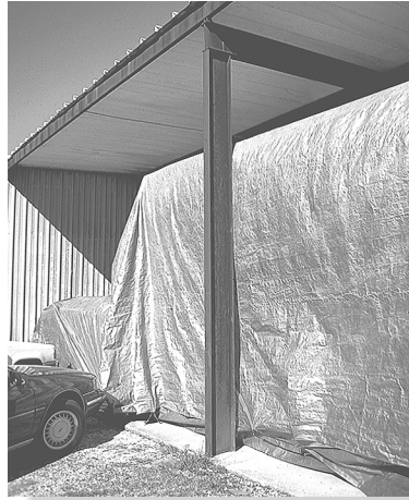
Wide-flange members are often used for columns. Here is an example of a beam column.
