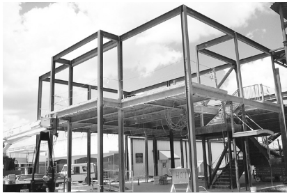
Typical steel framework.
